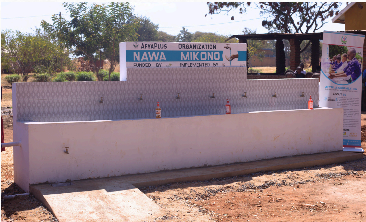
Newly Hand washing station constructed at Isimani secondary school in Iringa Dc
