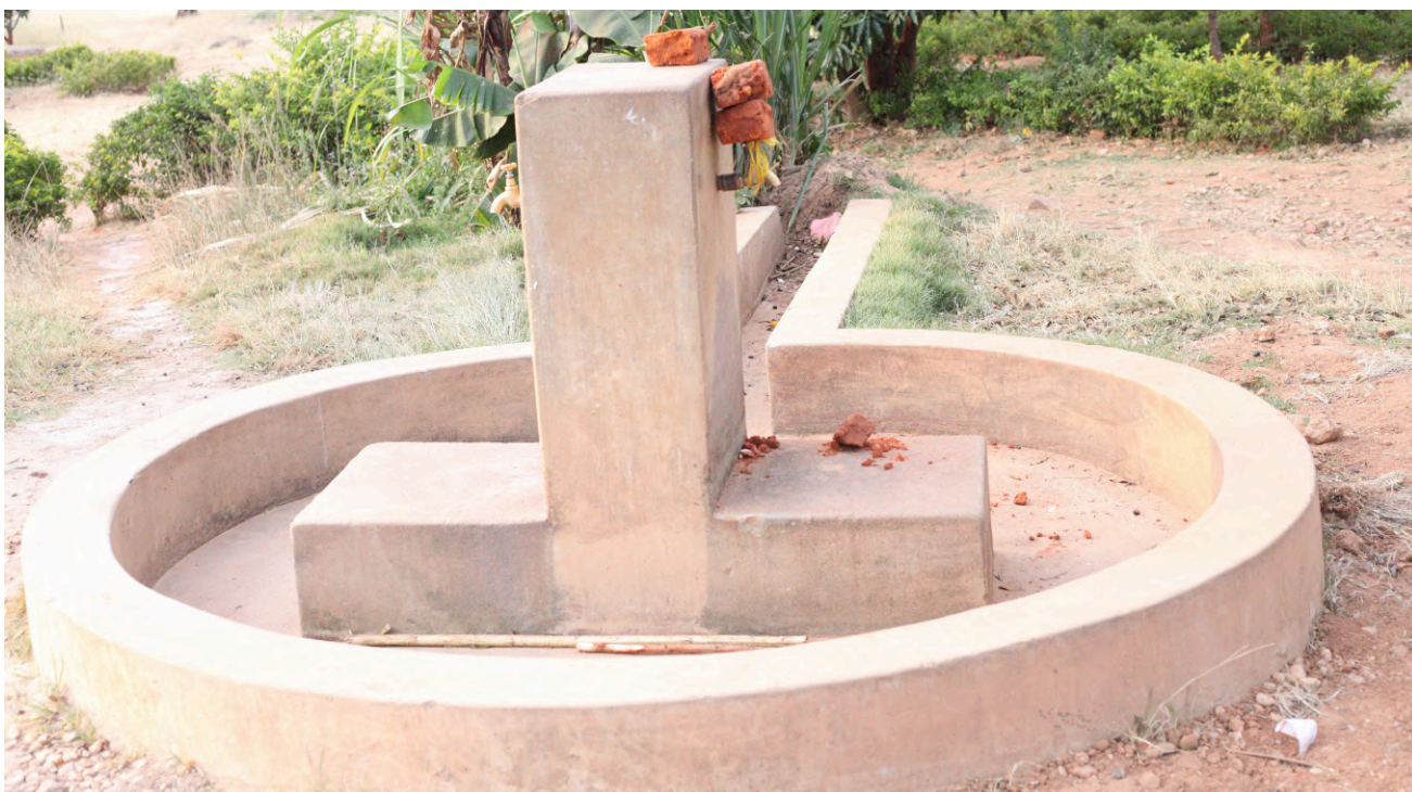
Hand washing station observed during the baseline survey. The station has two water taps, but only one is functioning, serving 681 students and other staff in the school.
