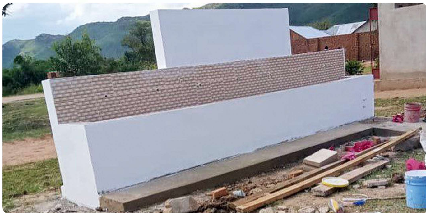
Implementation of hand washing facilities construction project at Mivinjeni Secondary.
