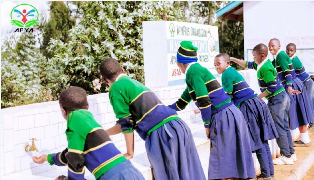
Figure 2: Hand washing facility constructed at Luhindo primary of Kilolo dc.
