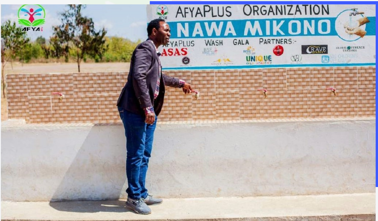
Fig 1. Afyaplus hand wash facility was constructed at Lipuli Sec of Iringa DC as a result of funds raised on
